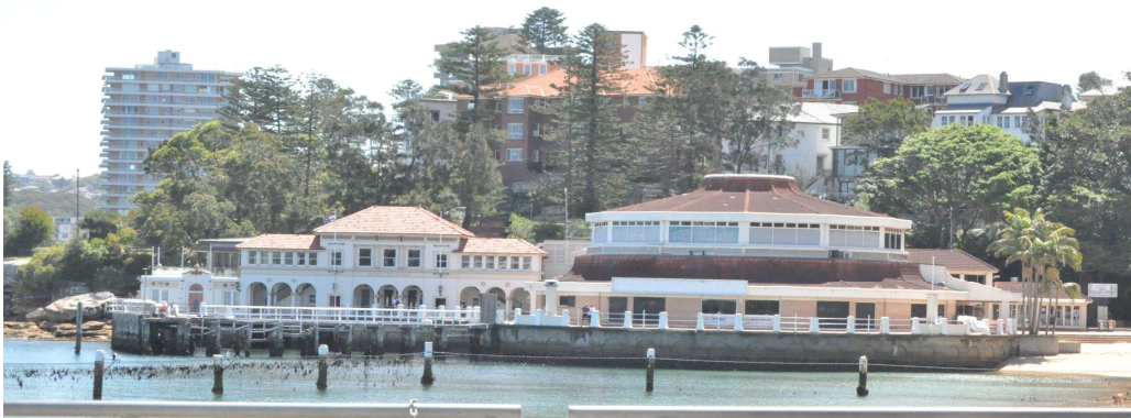
Figure 3: View of the existing former Sea Life aquarium building
